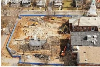
Aerial Photo of Demolition
