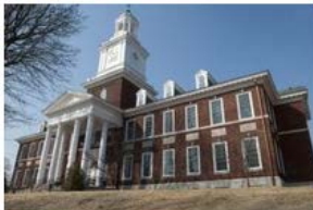
2010: Trickett Hall Renovation/Lewis Katz Hall Addition
